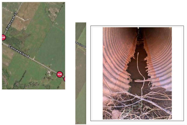
Conc 8 culvert # CLVRT00305
