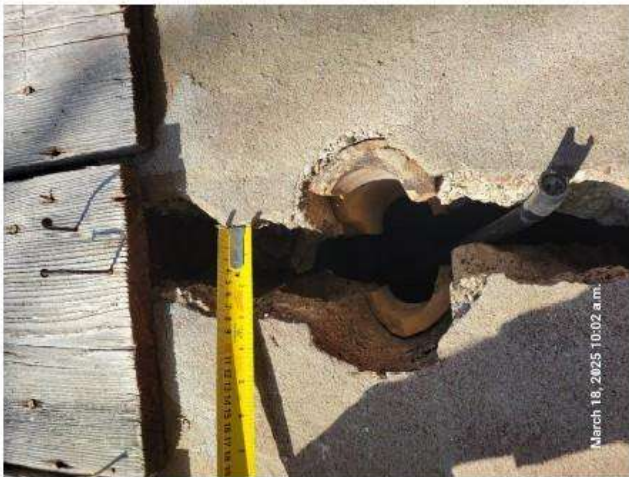
Severe crack in concrete foundation
